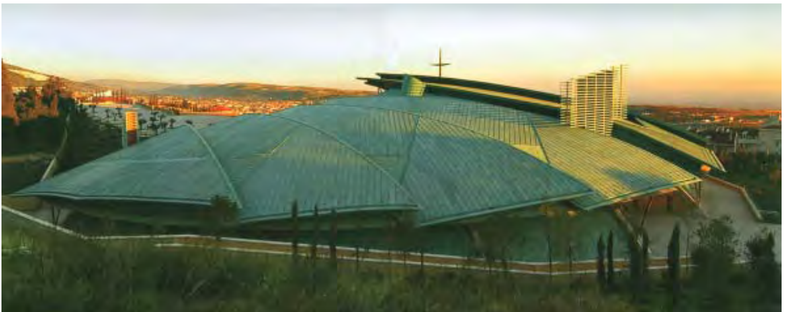
A rear view of the “new church” dedicated to Saint Padre Pio, in San Giovanni Rotondo (Foggia) - Italy.
